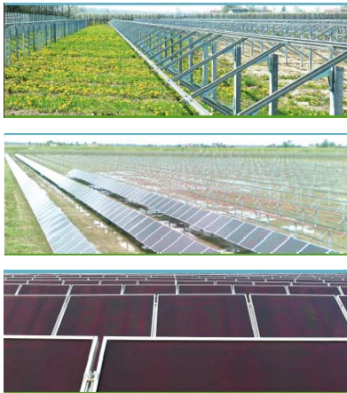
Carpi (MO) 680 kWp plant Amorphous silicon
